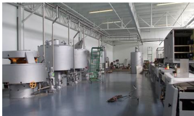
Figure 2. The TCHO factory floor under construction.
