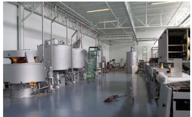
Fig. 2. A photo of the factory floor under construction.
